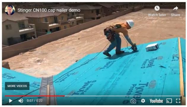
The product works fast. Its advertised speed is 5 cap nails per second, with a fastener capacity of 200 caps or nails. It reloads in less than 30 seconds and weighs less than five pounds. The CN100B marks an enhancement of the industry leading CN100 (shown above) and introduces an improved cap magazine for added durability.
