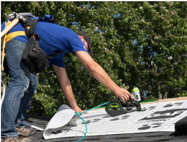
The newly-enhanced Stinger CN100B Cap Nailer in action.
